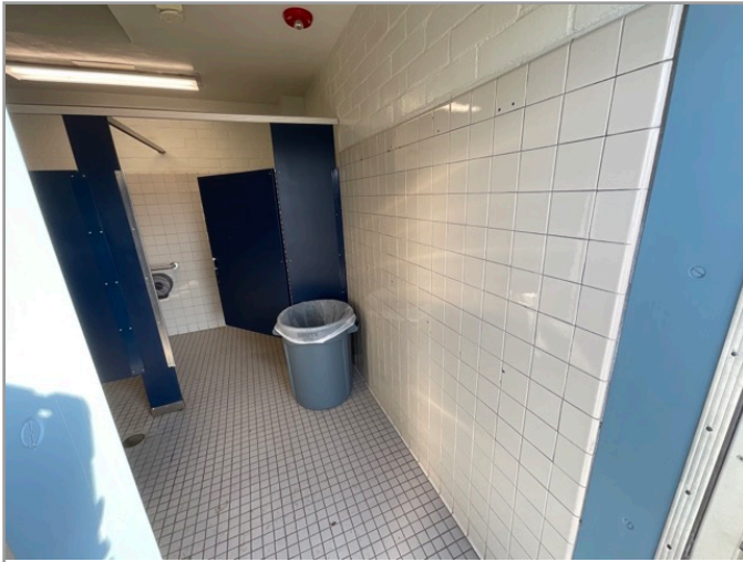
TOILET STALL OVERVIEW
