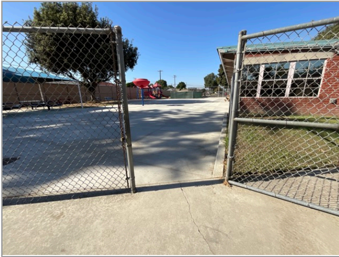
ACCESSIBLE ROUTE TO PLAYGROUND
