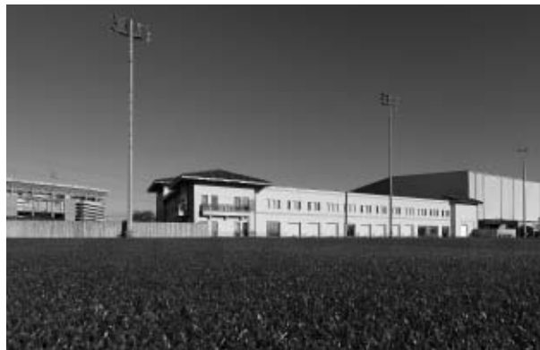
The facility features four 100-yard football practice fields as well as an indoor practice facility. On Sept. 9, 2002, LSU formally named its football practice facility for Charles McClendon, the winningest football coach in school history.
