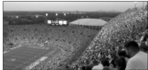
East Side Expansion of Tiger Stadium
