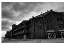
Combined HDR image
