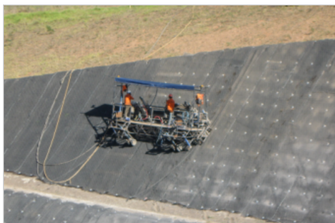
Installation crew drilling and grouting bolts
