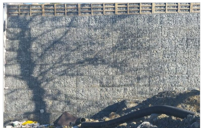
12m High Terramesh Wall Under Construction
