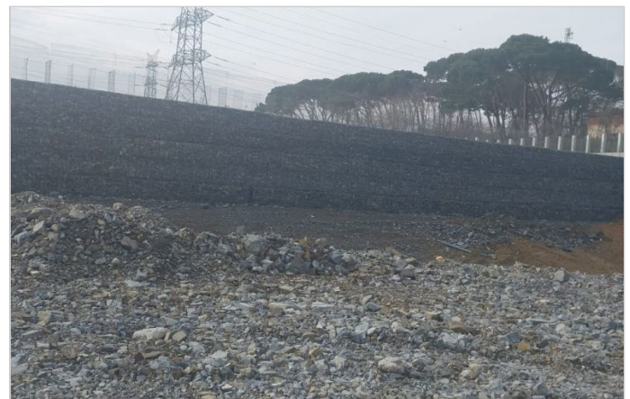
Terramesh Wall Supporting the Football Field
