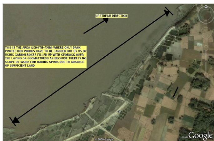
Photo 2: Eroded riverbank before construction
