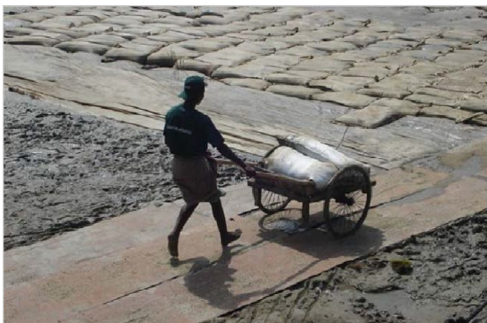
Photo 5: MacBag® being carried in a wheel barrow for placement
