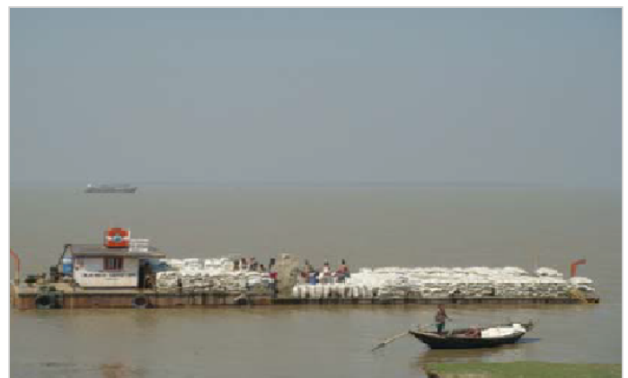
Photo 6: Stacking and filling of MacBags® on the barge and dumping of bags
