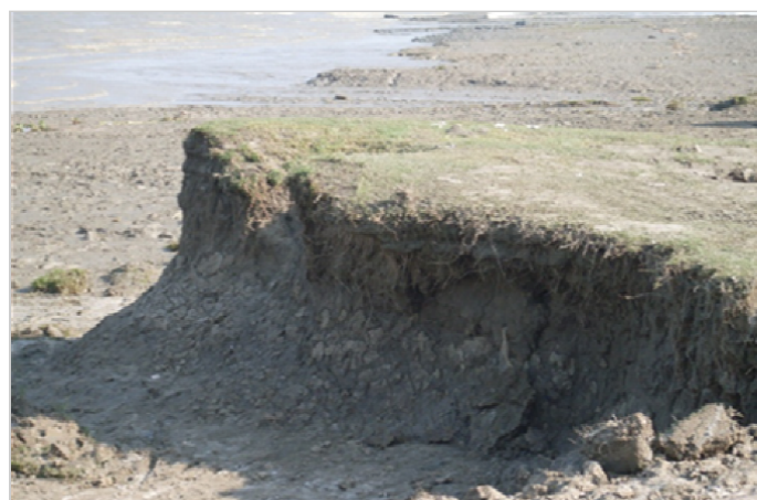
Photo 1: Site eroded due to wave effect
