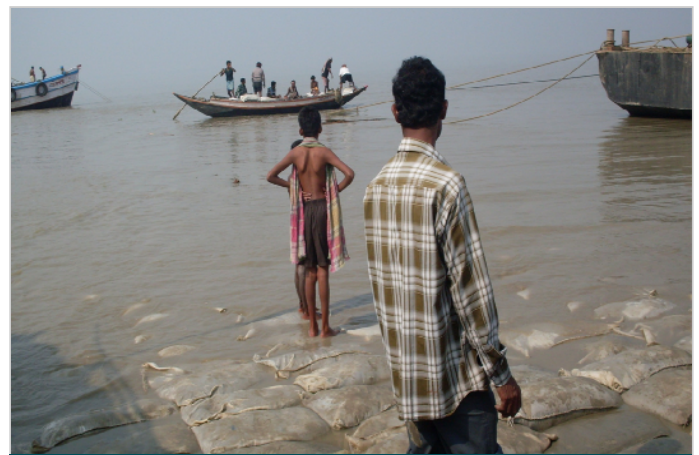
Photo 4: Placing of MacBags
