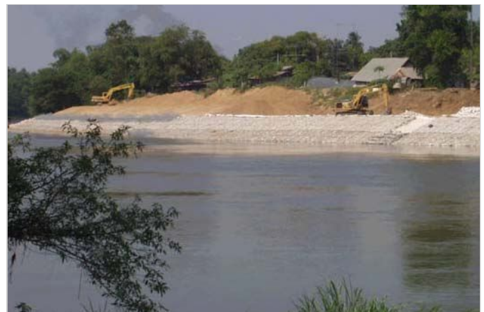
During Reno Mattress installation (1)
