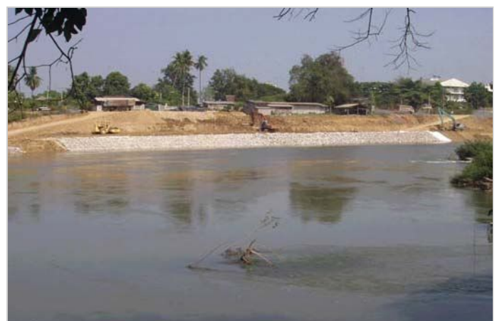
During Reno Mattress installation (2)
