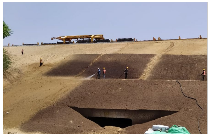
Photo 2: Application of MacGanics
