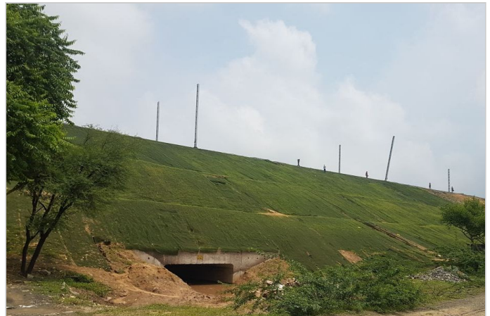
Photo 6: Vegetation establishment on slopes installed with MacMat
