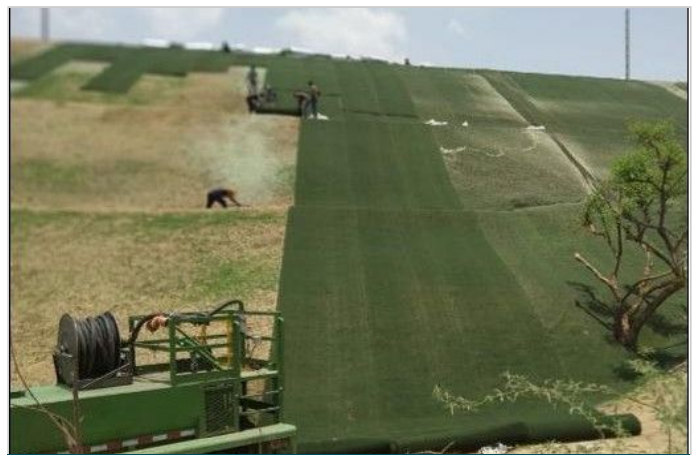
Photo 4: Laying of MacMat and fixing of U-pins over HECP surface
