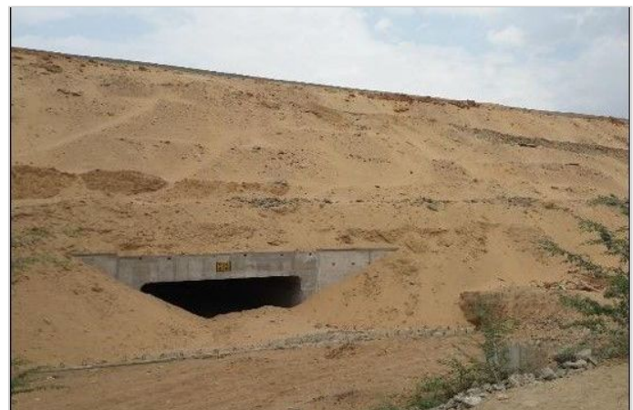
Photo 1: Site before application of erosion control products
