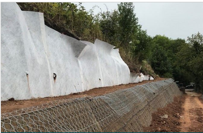
Macdrain was used to the rear of the reinforced soil to
