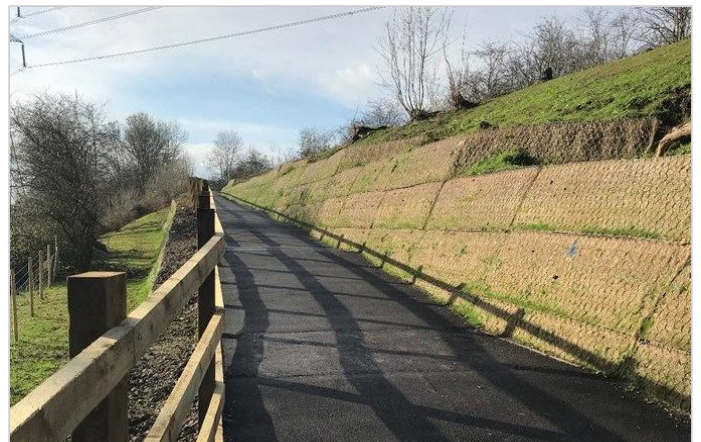
Completed upper Green Terramesh slope &
