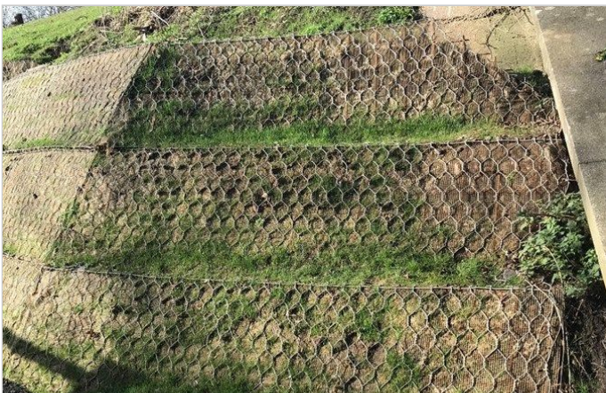
Stepped corner return detail tying into bridge
