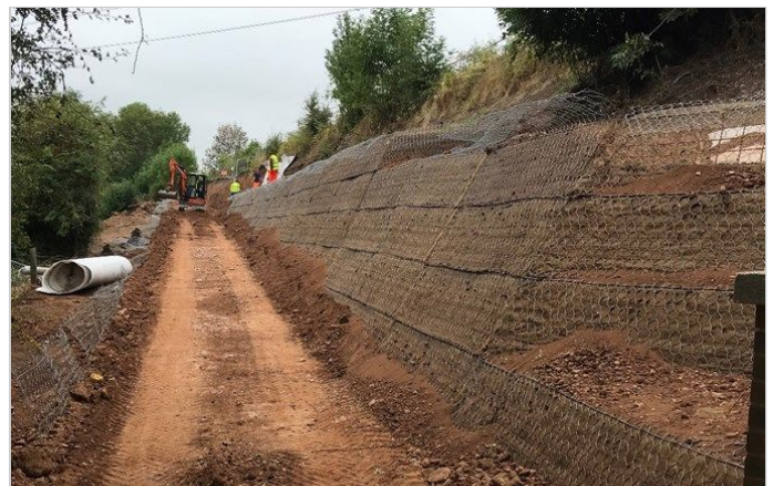
Construction of split level Green Terramesh to form
