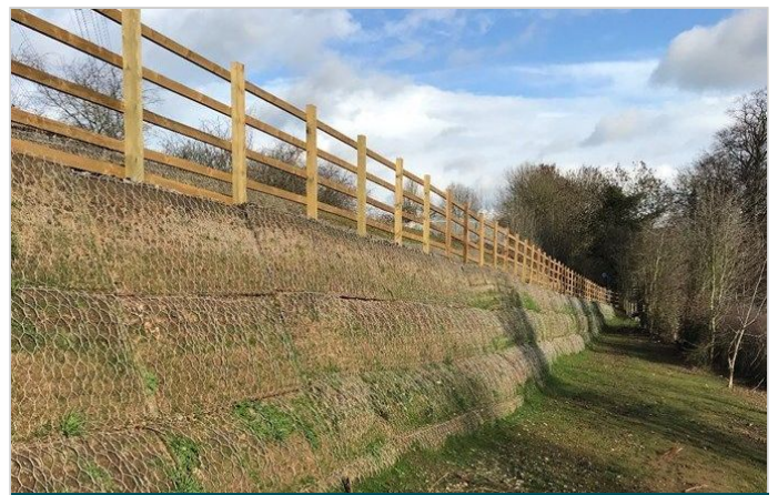
Completed lower Green Terramesh slope starting to
