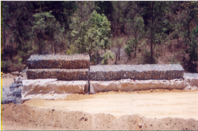
Photo 3: Gabions filled with rock and geotextile underneath
