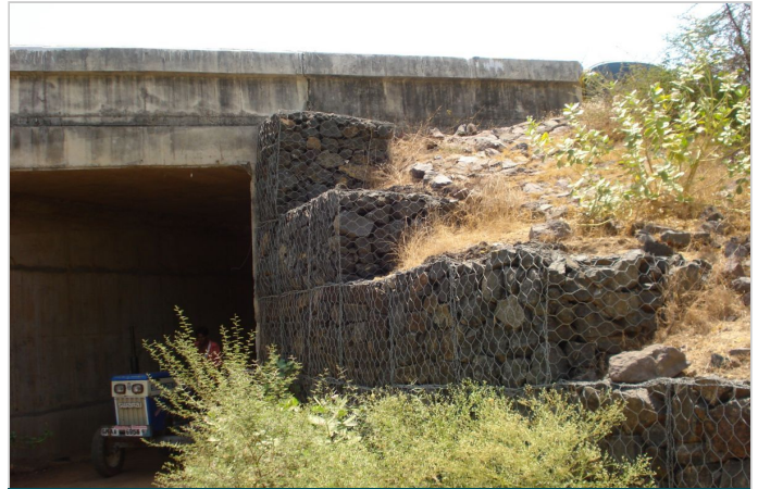
Photo 4: Completed gabion wall for culvert protection
