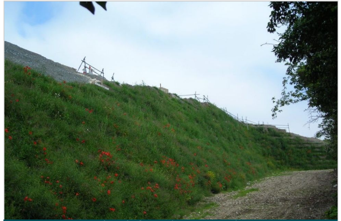
Green Terramesh reinforced vegetated
