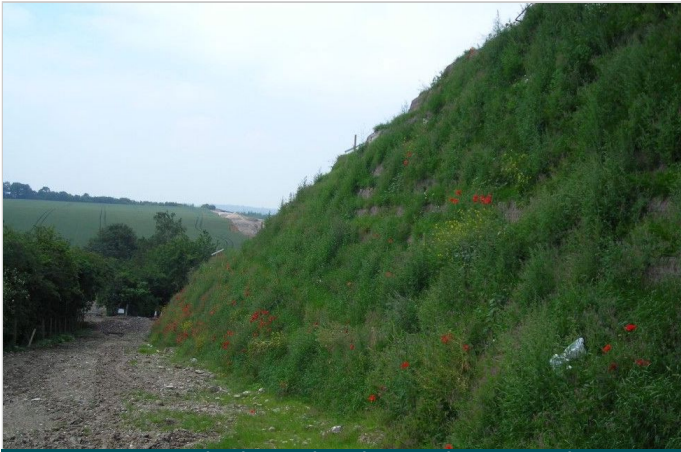
Green Terramesh slope showing early vegetation
