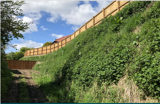
Green Terramesh structure complete and vegetation establishing well
