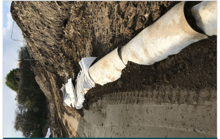
MacDrain installed between reinforced soil block & existing soil
