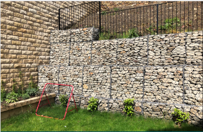
Gabion walls between plots
