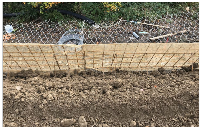
Green Terramesh - note factory-fitted braces and face support
