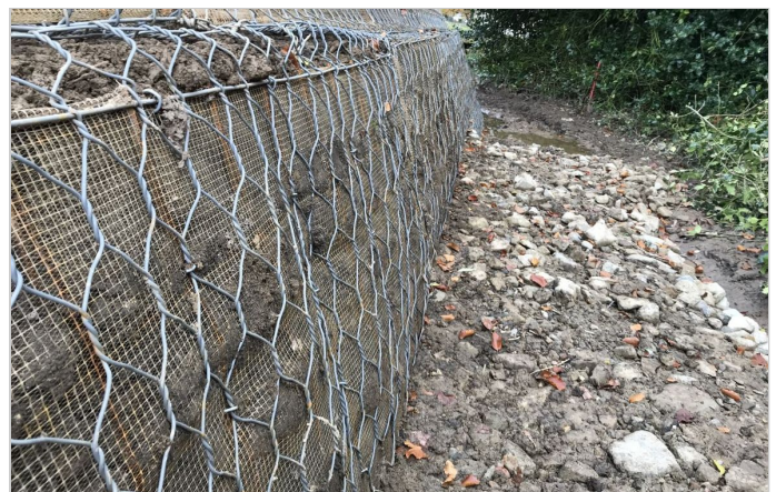
Green Terramesh unit erected - no external formwork
