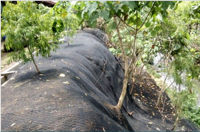
June 2016 - Complete Installation of MacMat R for Erosion Control
