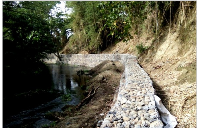
June 2016 - Complete Installation of Gabions as Toe Wall
