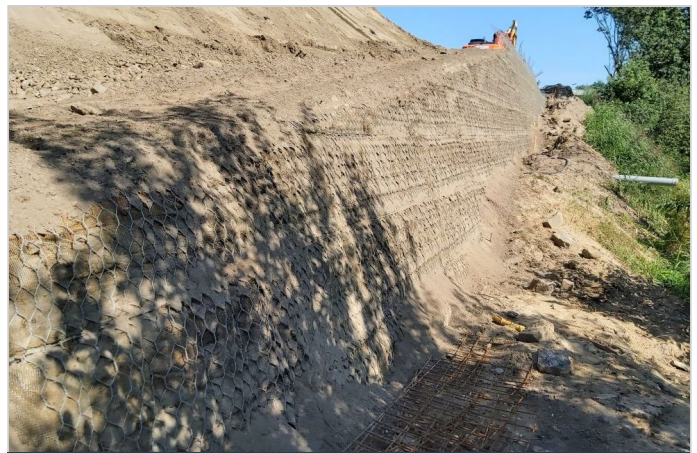
During the installation
