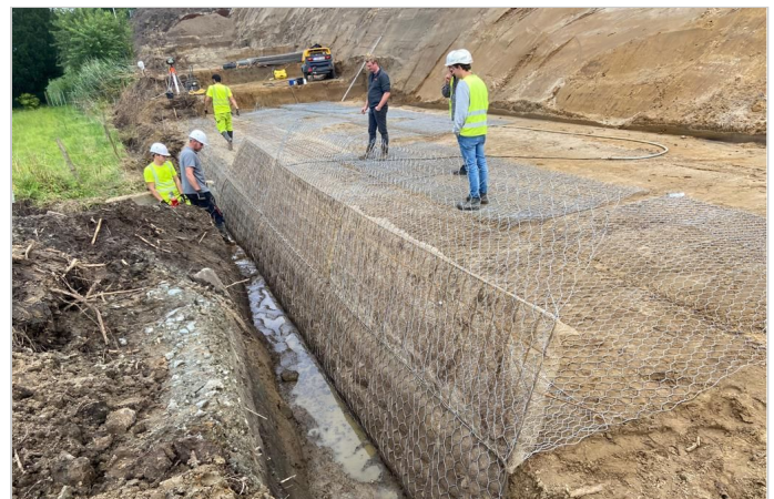
Start of the installation phase
