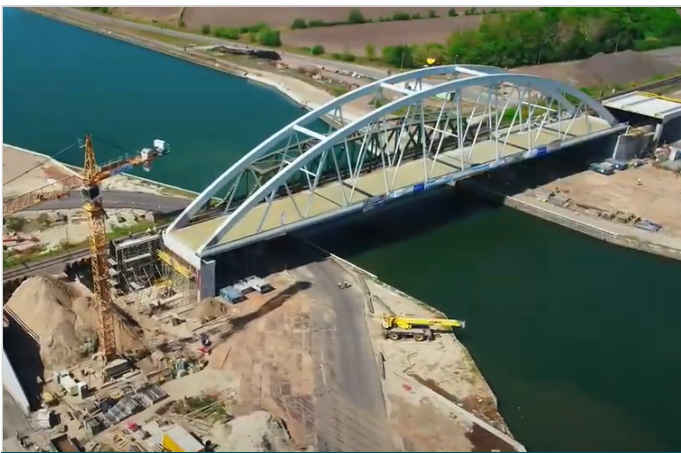
Bridge arch positioned
