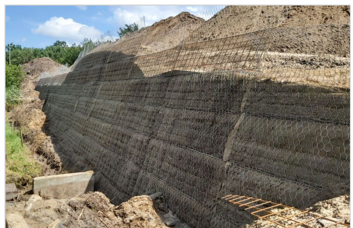
During the installation
