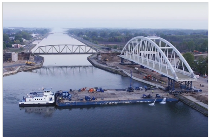
Bridge arch before the positioning phase
