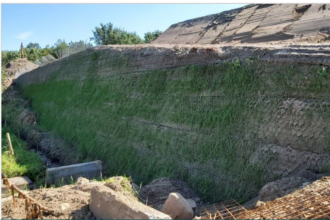
Construction phase: side view detail
