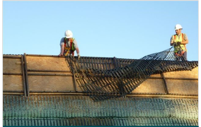
Wrapping Paragrid geogrid back to form face of bund
