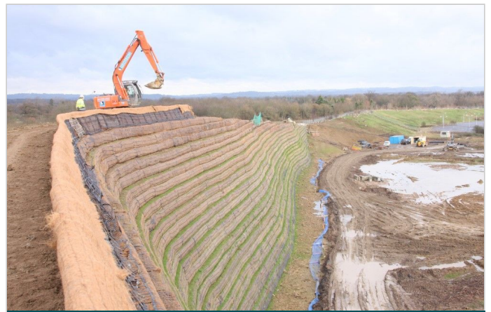
The bund nearing full-height
