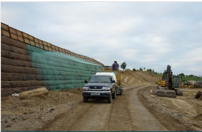
Hydroseeding the bund during construction
