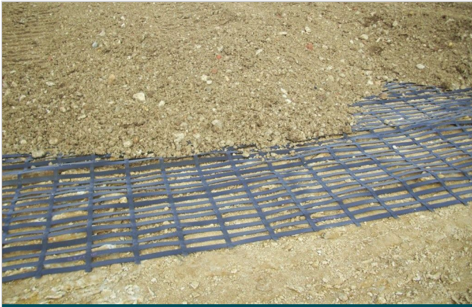
Recycled granular fill was used at the base of the bund
