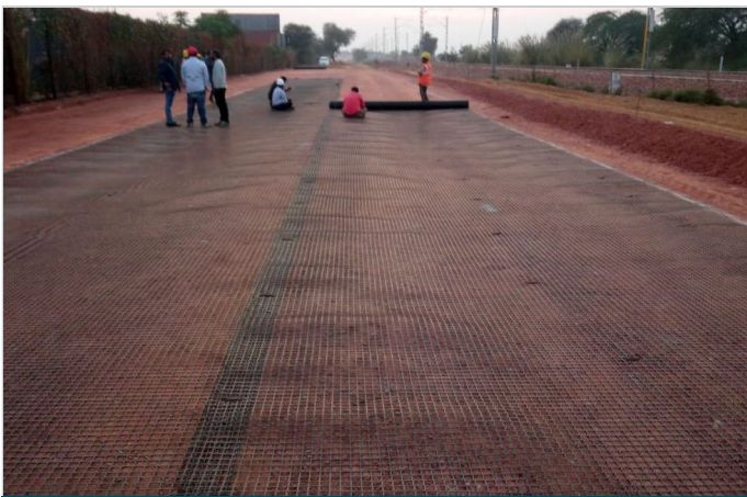
Photo 4: Installation of MacGrid EG Geogrid
