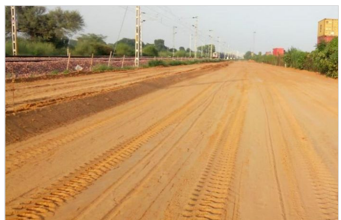
Photo 2: Site during construction
