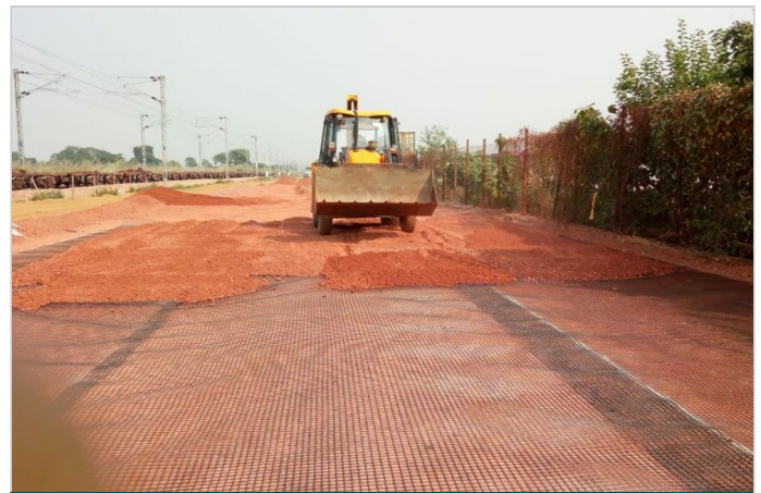
Photo 6: Laying of Blanket layer over MacGrid EG
