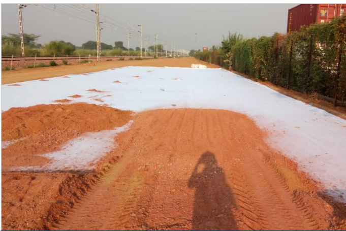
Photo 3: Laying of MacTex Geotextile and Blanket layer
