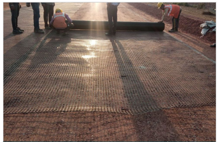
Photo 3: Unrolling of MacGrid EG Geogrid
