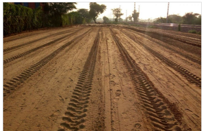
Photo-1: Site during construction
