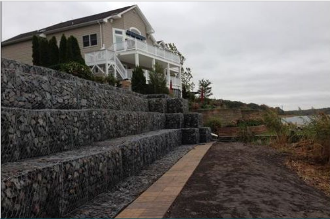
Post installation- completed wall
