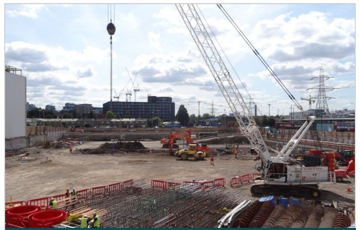
Working platform prepared to support the CFA rig
