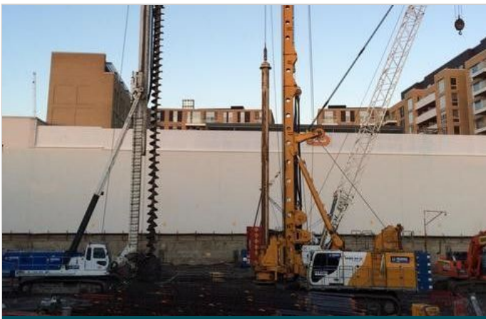
During final works - September 2015
