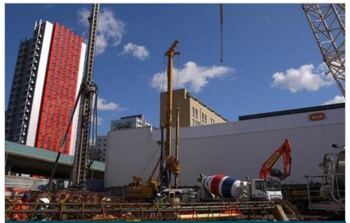
General view of the site from Silvertown Way
