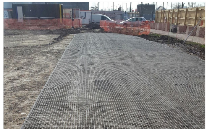
Installation of MacGrid WG on first phase (AREA 1)
