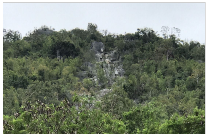
Source of Rockfall (Photo Taken From Road Level)
