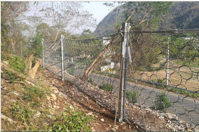
Rockfall Barrier Completed Installation
