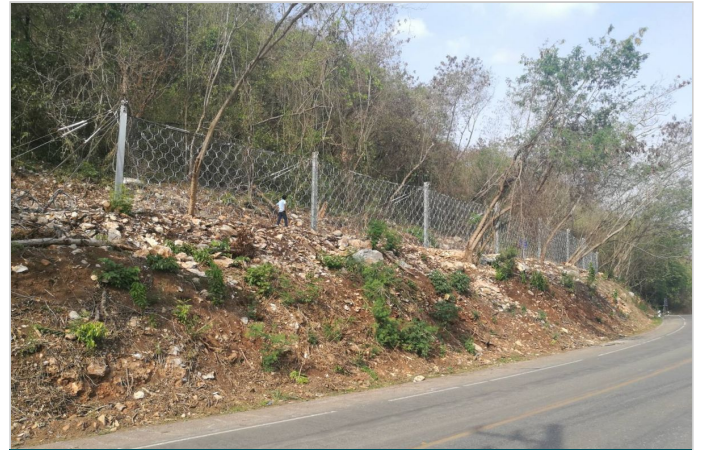
Rockfall Barrier Completed Installation
