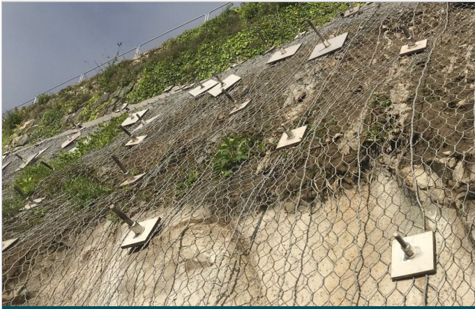
Steelgrid HR 30 PVC secured to the embankment
