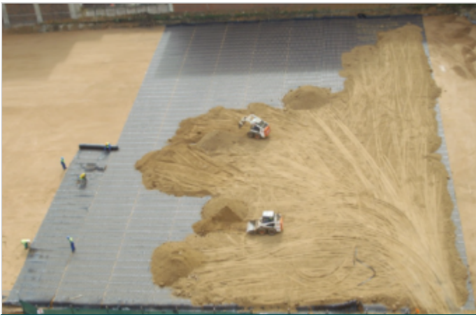
The contractor laid and covered up to 5000sqm of Paralink™ per day and was only
