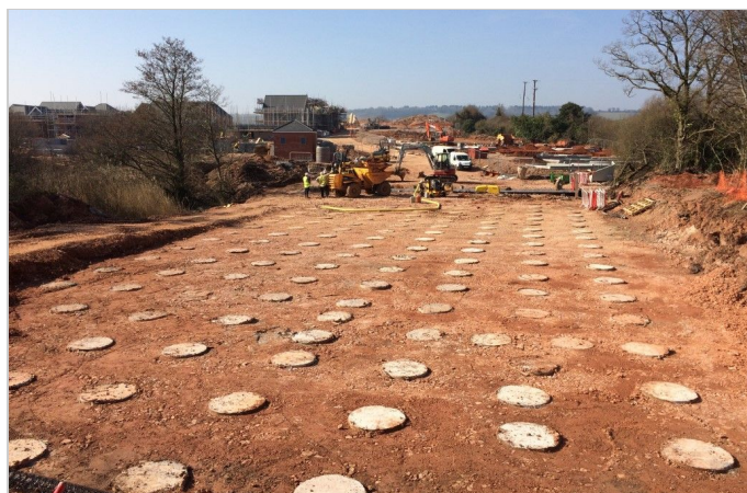
Global view of the site - Piling configuration
