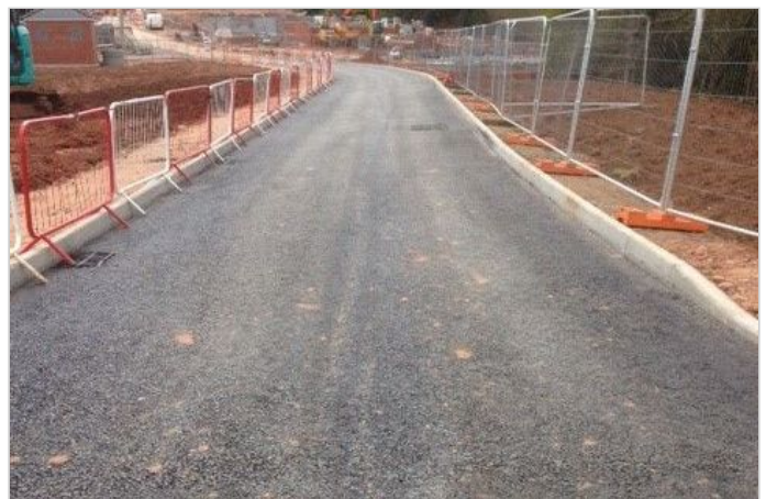
Finished surfacing on the road
