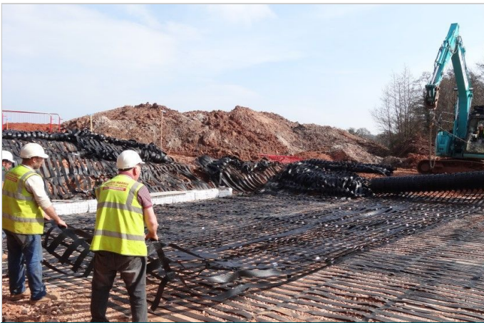
Installation of the transversal layer of ParaLink®
