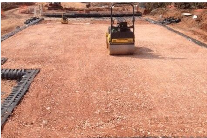
Final compaction operation for the basal reinforcement
