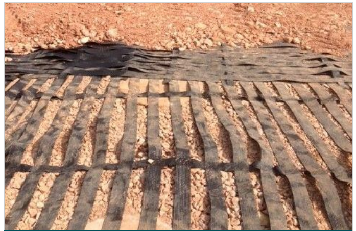
Layers of ParaLink® within compacted 6N material
