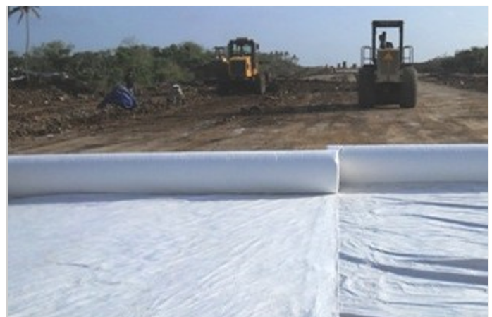
February 2011 - During Construction - Laying of Non-woven Geotextile
