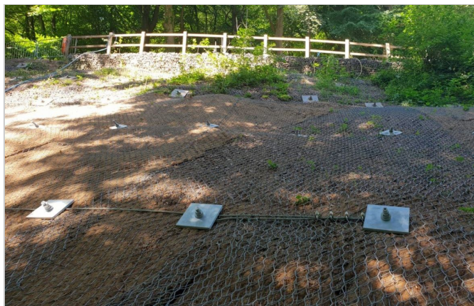
Steelgrid HR in place stabilising the face of the embankment
