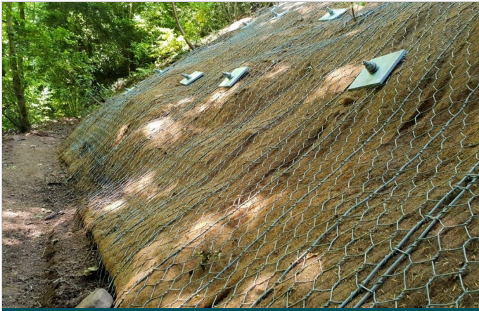
Soil nails and Steelgrid HR
