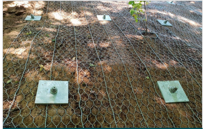
Steelgrid HR system securely in place, with vegetation starting to establish
