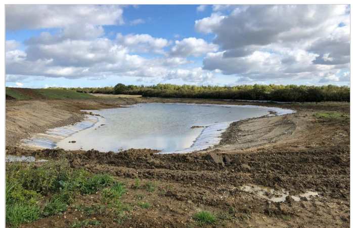
MacLine GCL lining in place post-construction
