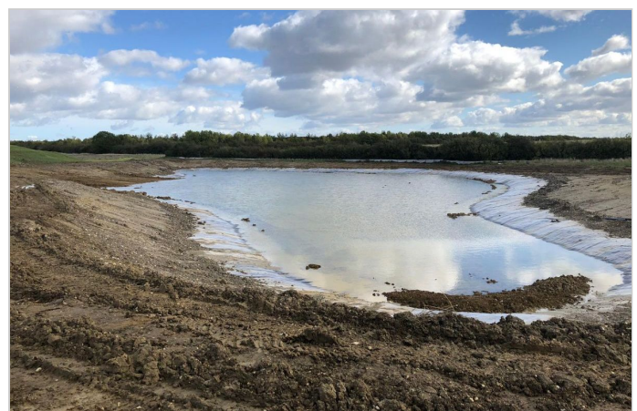
MacLine GCL lining in place post-construction
