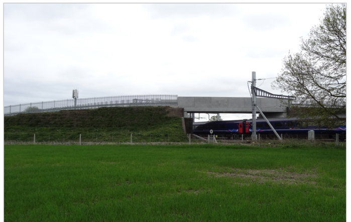
Green Terramesh® ramps vegetated in April 2018
