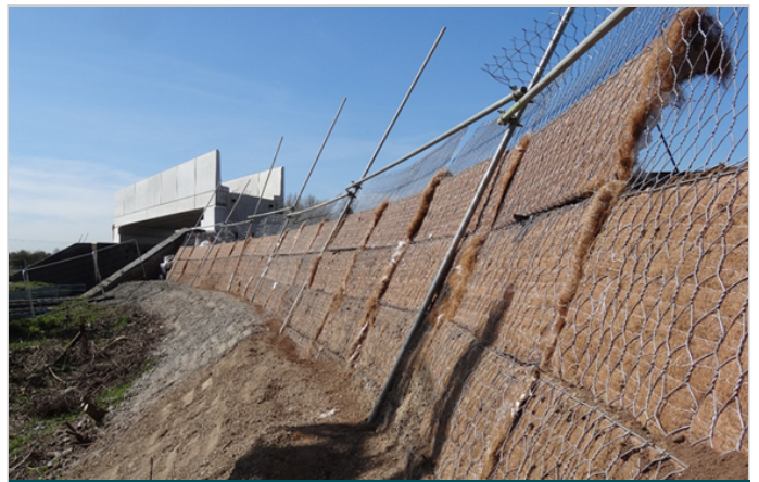
Fourth course of Green Terramesh® being placed on the North ramp
