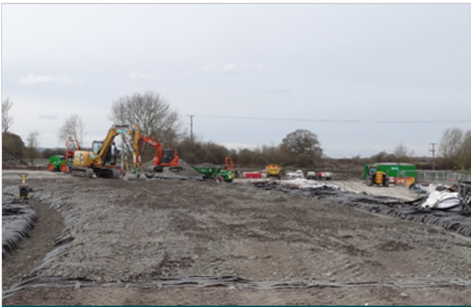
Paralink placed over soft soil and wrapped back in an anchor trench
