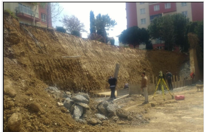
Excavation of the foundation
