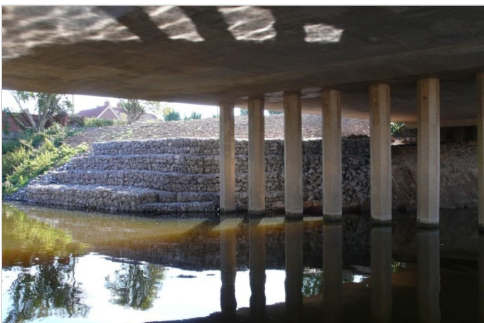
PA6 gabion bank protection complete in August 2016
