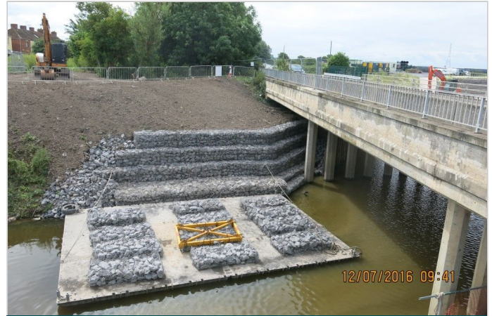
General view during construction - July 2016
