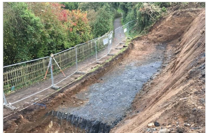
Area for Green Terramesh footing cleared and prepared
