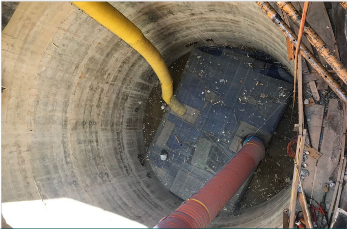
Shaft area protected using RockMesh3030
