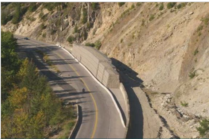
Completed Structure, August 2008
