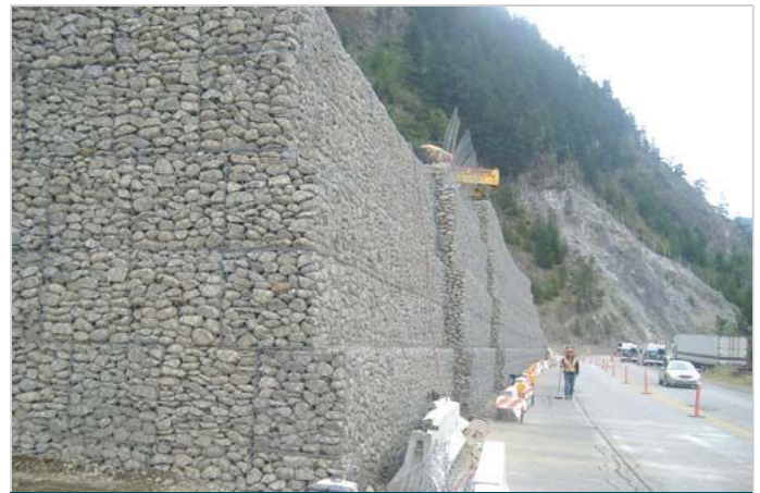
Completed North End of Structure
