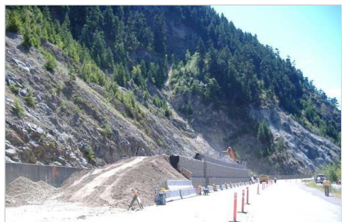
North End Access Ramp During Construction
