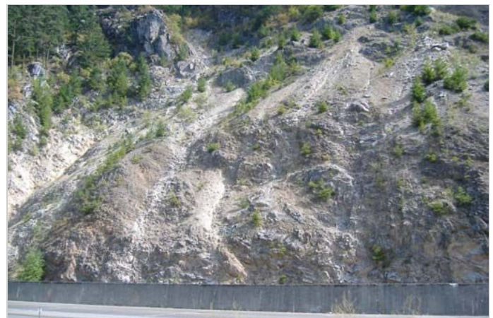
August 2008 Existing Concrete Barrier Wall and Rock Slope Conditions
