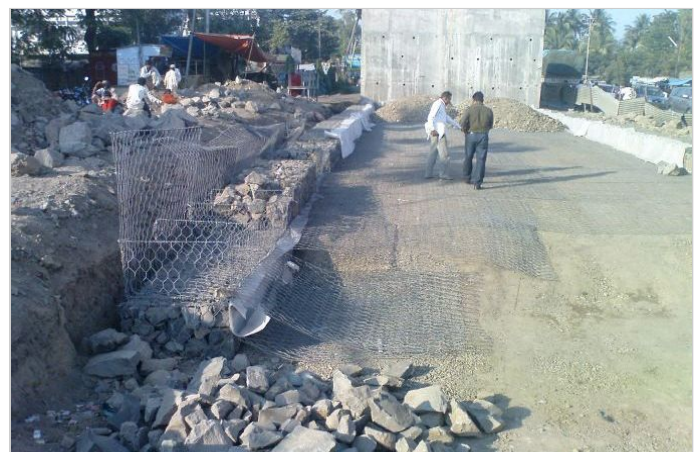
Photo 1: During construction - Filling TMS units
