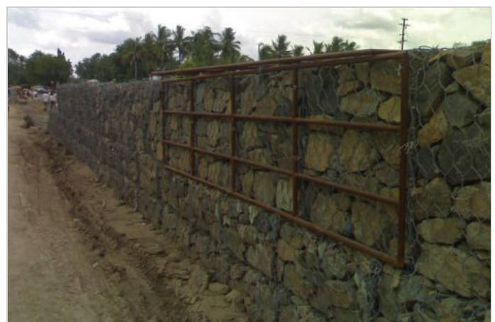
Photo 2: During construction - Checking vertical
