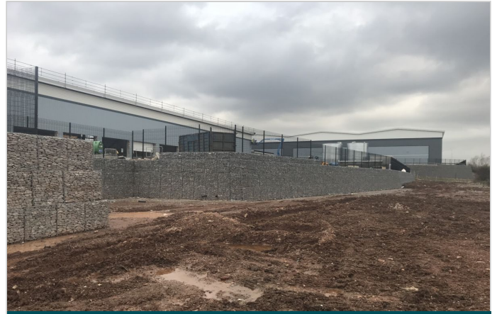
Walls at DPD location completed - the total length of the wall is 220m
