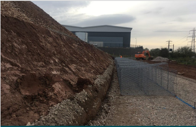
Gabion set out at DPD development location - Autumn 2017
