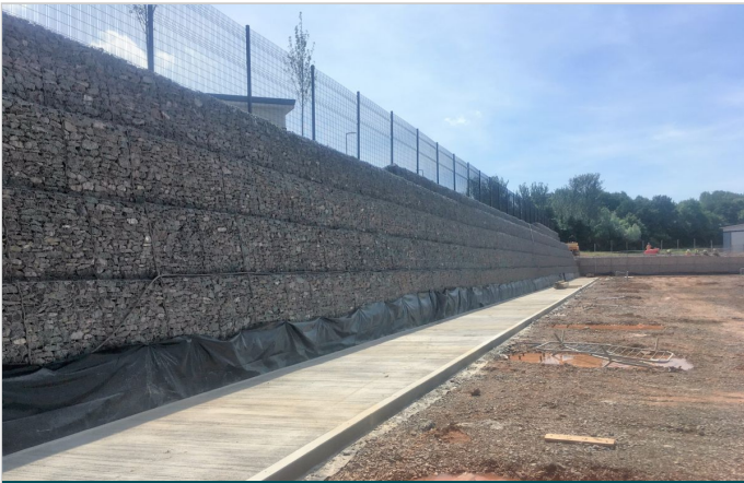
The Terramesh wall at Geary's Bakery location is 100m long by 4.5m high
