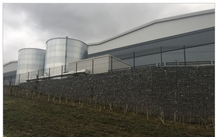
Water tanks behind the wall were placed over a concrete slab.
