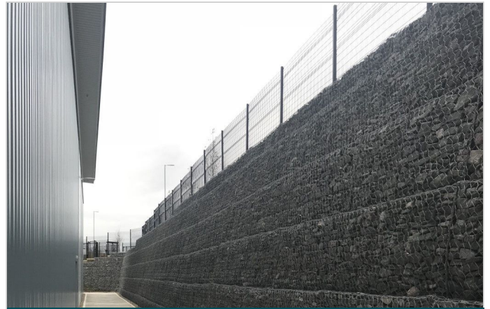
Terramesh System installed at Geary's Bakery
