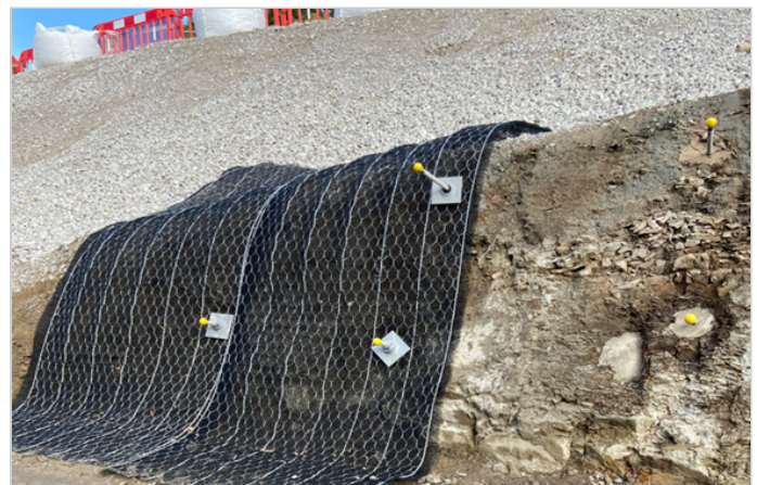
MacMat HS30 P being installed on the rock slope.
