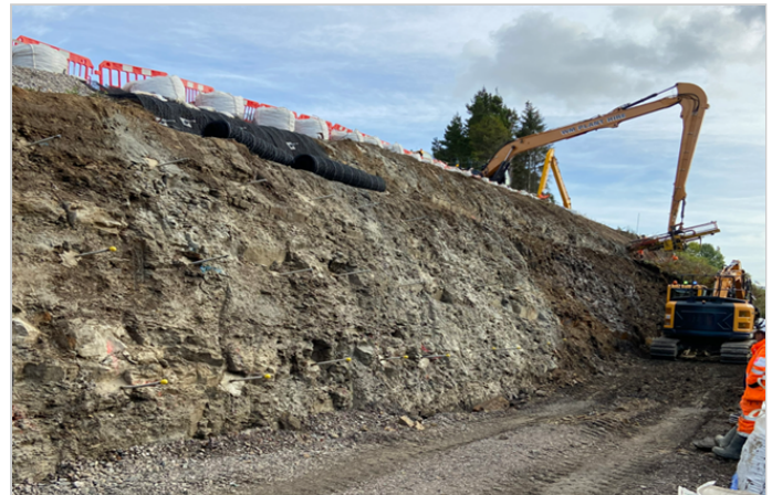
Soil nailing of the newly cut rock slope adjacent to the rail line.
