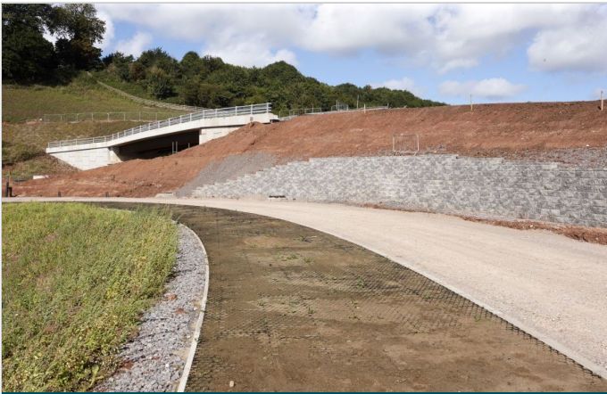
MacWall construction moving forward towards completion
