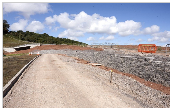
Slip road with further construction of MacWall
