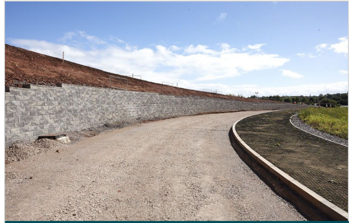
Slip Road Section - MacWall Vertica - 4 Degrees BBA
