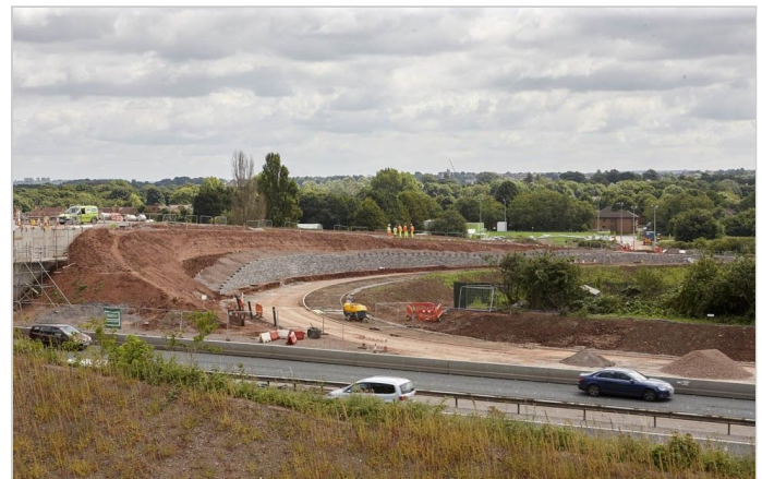
MacWall construction with reinforced soil support
