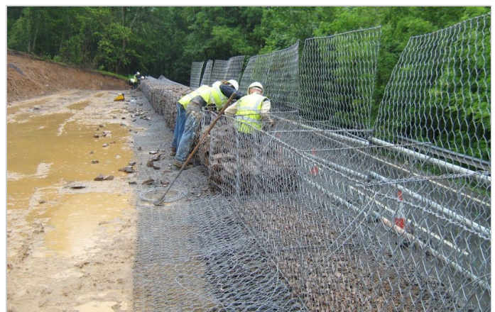
Filling of integral gabion facia
