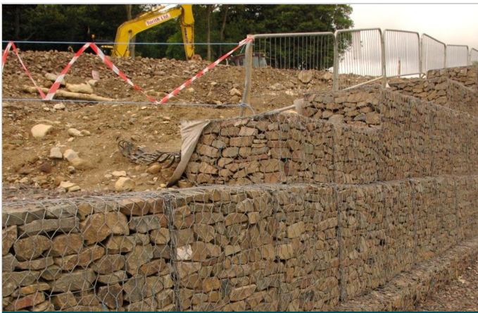
Completed Terramesh® units
