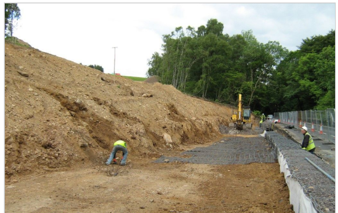
Installing Terramesh® soil reinforcement
