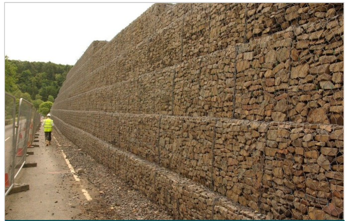
Completed structure with highway above wall
