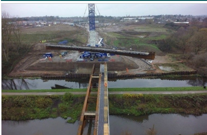
Crane pads over CFA foundation piles.
