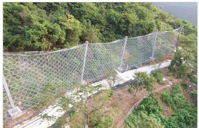
Complete installation of dynamic barrier (aerial view)
