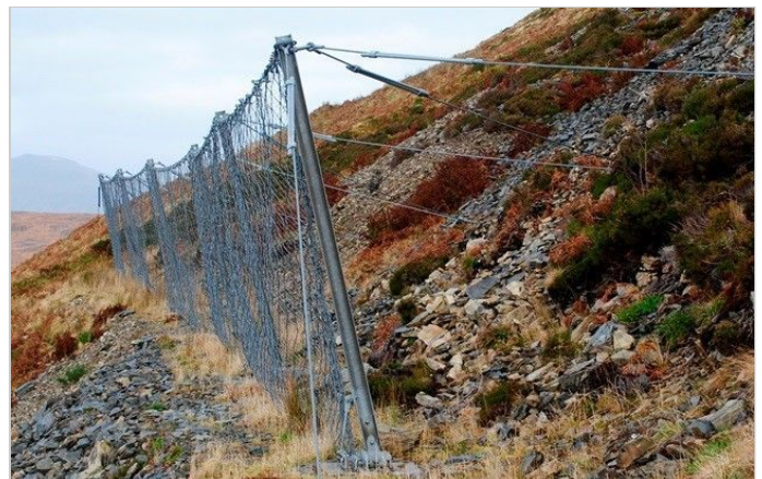
Dynamic barrier condition in 2014 (view N) after 5 years on-site
