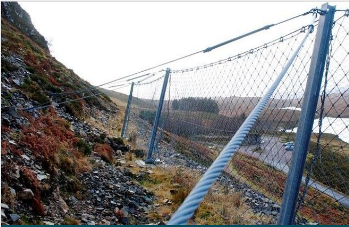
Dynamic barrier condition in 2014 (view S) after 5 years of use
