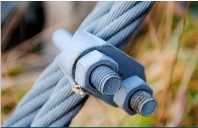
Galvanised rope grips showing very slight surficial corrosion (2014)
