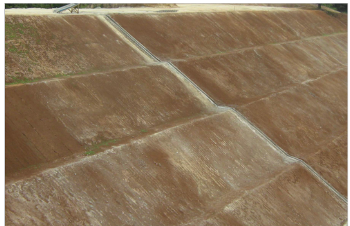
March 2009 - During Construction
