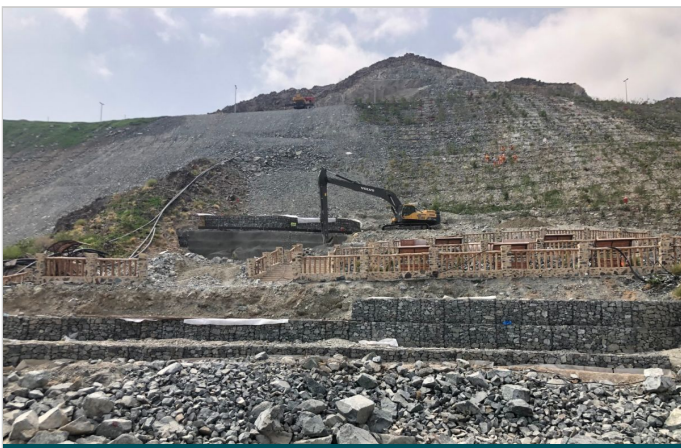
Installation of Terramesh core in progress
