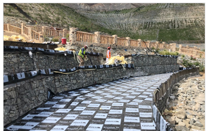
Installation of Terramesh core in progress
