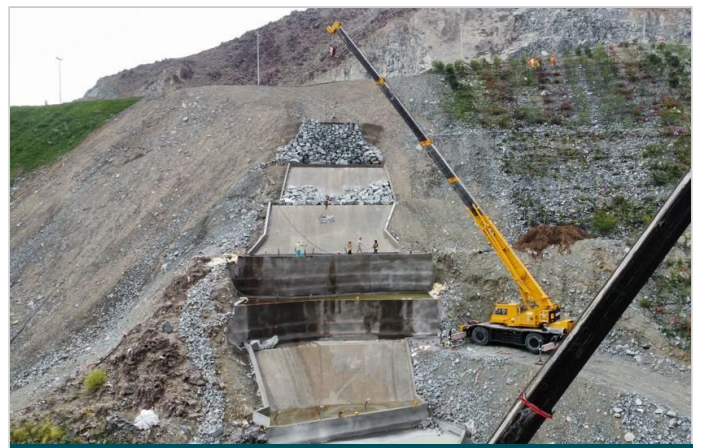
Applying of gunnite concrete cover in progress
