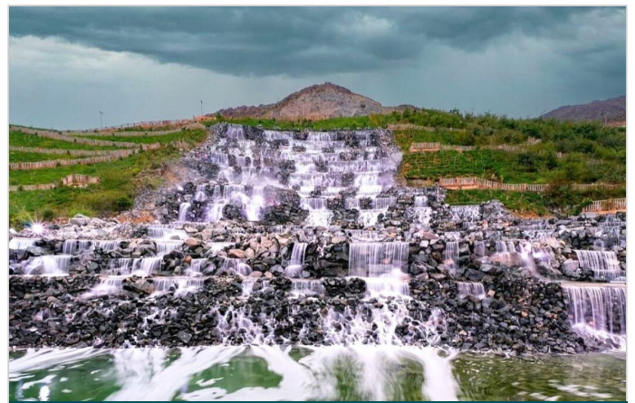
Completed project: Close view of Cascading Waterfall
