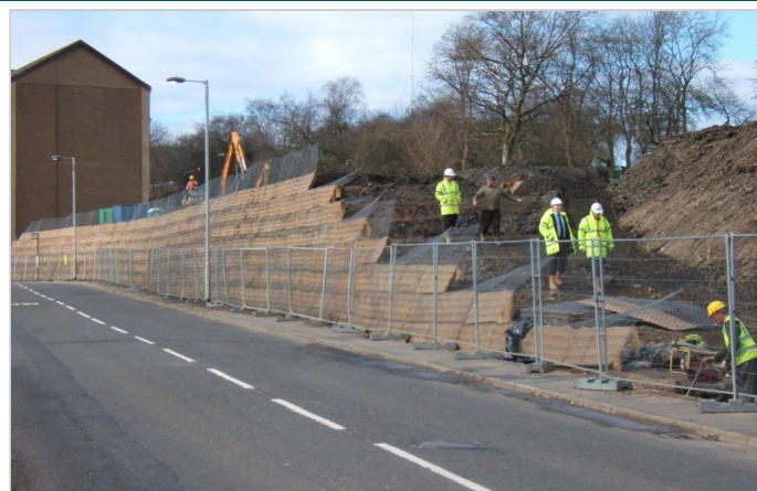
Structure nearing completion
