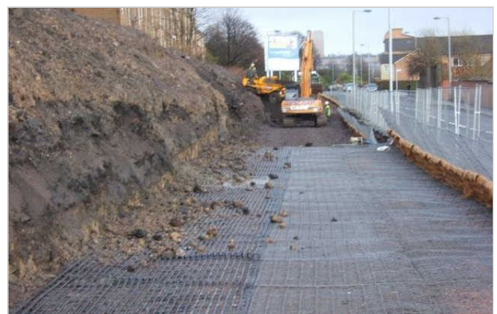
Green Terramesh® geogrid installation
