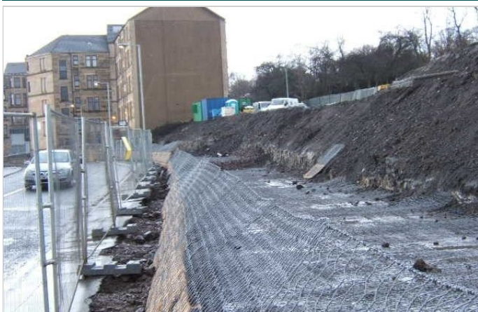
First Green Terramesh® layers being installed
