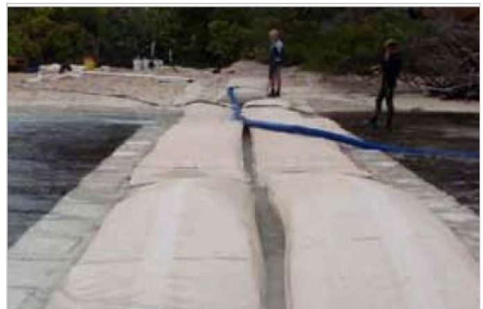
Installation of top row of MacBags on groin
