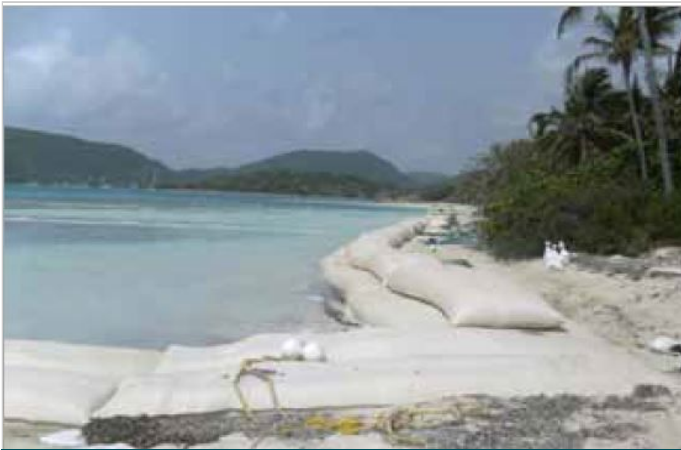
Revetment and groin with MacBags during construction
