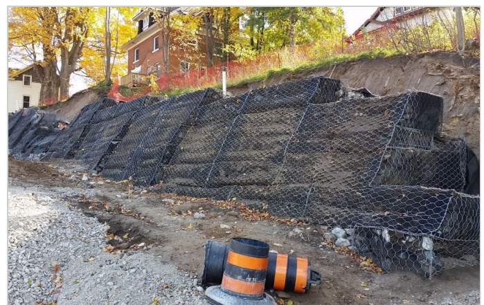
Green Gabion Wall during installation
