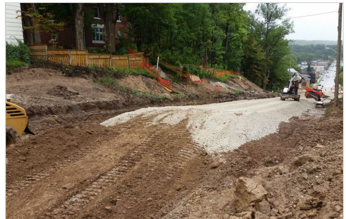
View of original slope before construction of the wall
