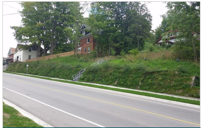
Downhill view of finished wall
