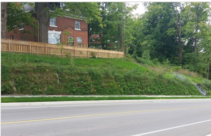
Uphill view of finished wall
