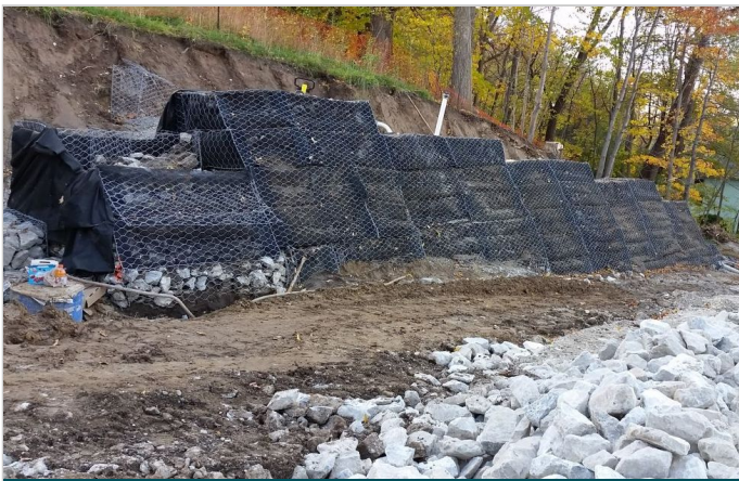
Detail of Green Gabion Wall units
