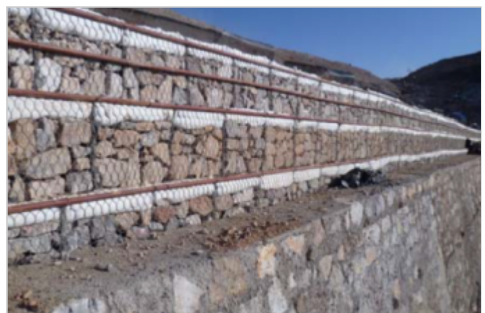
Terramesh gabion fascia units - optional temporary formwork
