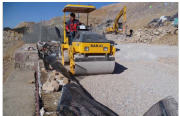
Preparing the foundation to the Terramesh wall
