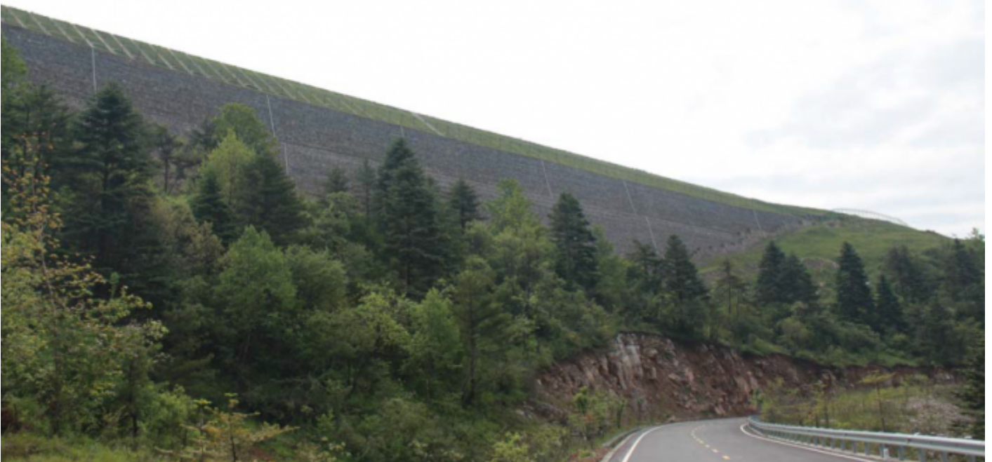
Completed Terramesh structure supporting runway
