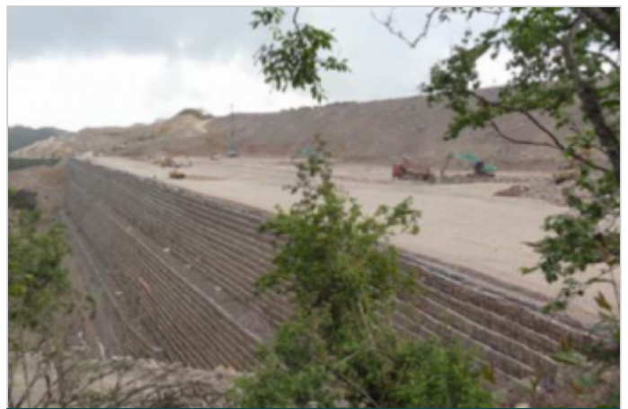
Reinforced soil wall under construction
