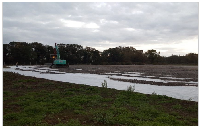
MacTex W2 laid over the existing ground - Oct 2015
