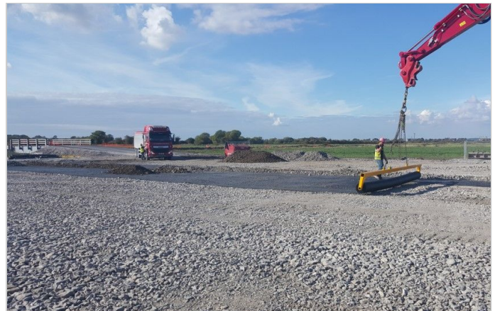
MacGrid WG laying operation using a spreader bar
