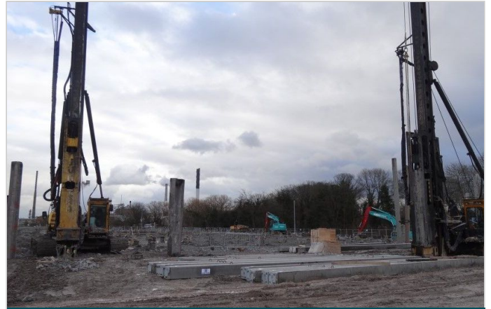
Junttan PM20 machines during final operation in Jan 2016
