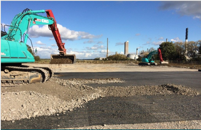
Placement of granular material (in this case, Class 6F5 GMA)
