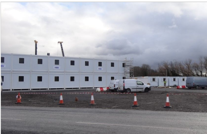
Soil stabilisation using MacGrid WG in the compound/tracking areas
