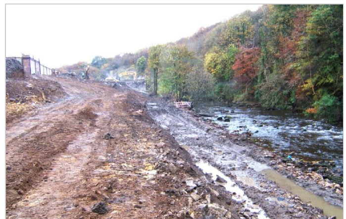
Downstream view of prepared slope
