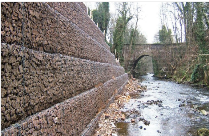
Post-construction restored bank protection
