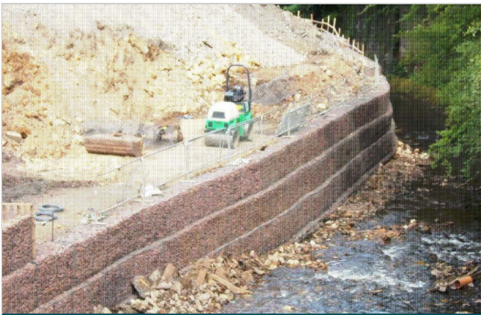
Upstream view of Terramesh wall during construction
