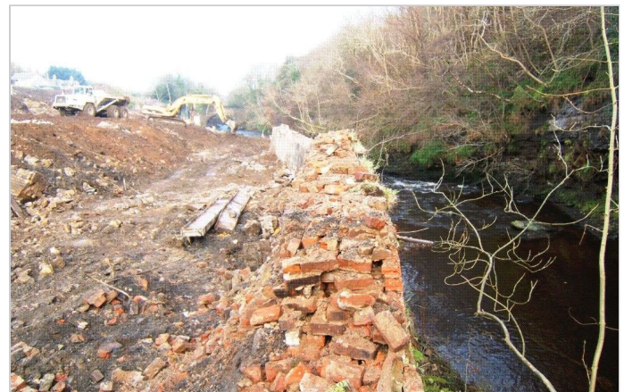
Existing masonry wall before construction
