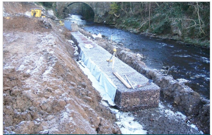
First course of Terramesh during construction
