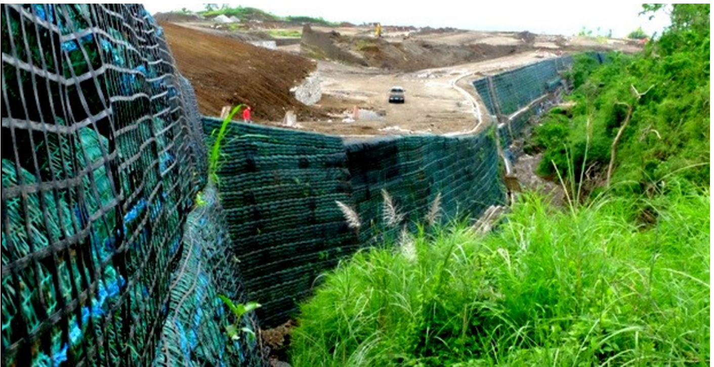
August 2016- Project Near Completion
