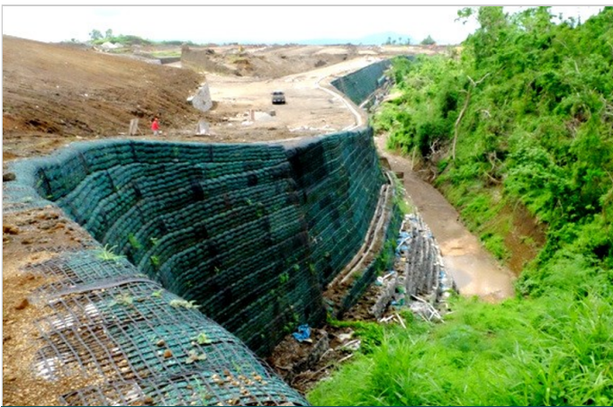
August 2016- Project Near Completion
