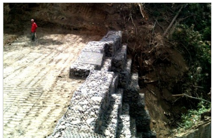
January 2014 - During Construction
