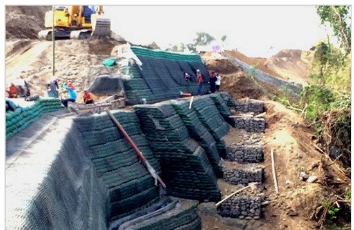
January 2014 - During Construction
