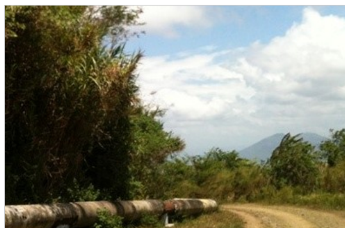
March 2014 - Existing Site Condition
