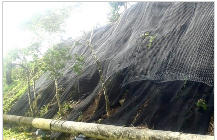
October 2014 - During Construction
