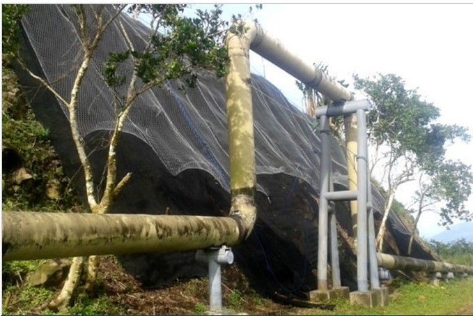
October 2014 - During Construction
